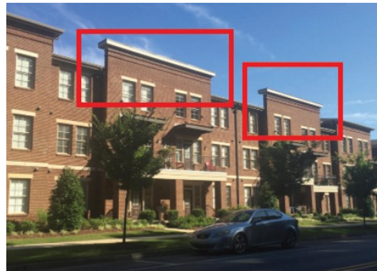
Figure 1117-D: Example of a cornice (left image) and parapet (right image), both highlighted in the red rectangles.
