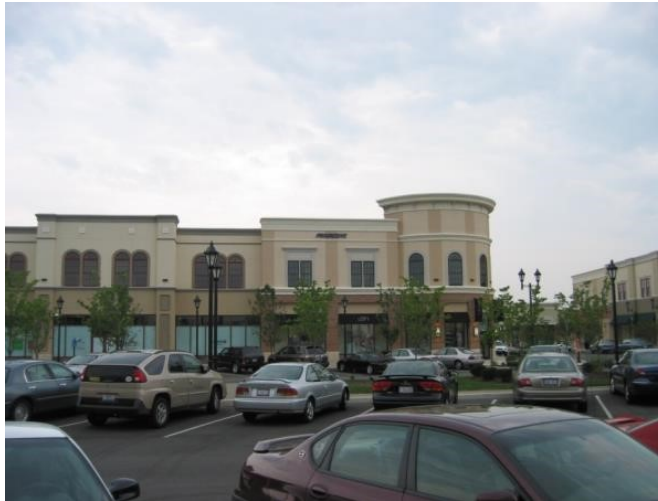
Figure 1117-I: Roofline changes shall be aligned with corresponding wall offsets and/or material or color changes.
