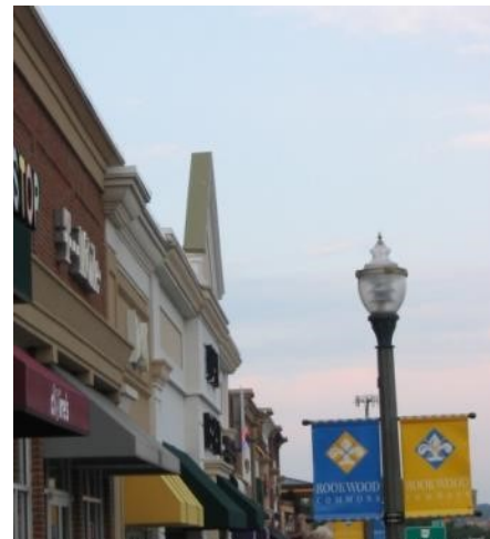
Figure 1117-J: Parapet walls with cornice treatments are used to disguise flat roofs. The image on the right illustrates a tall, thin parapet wall that is prohibited.
