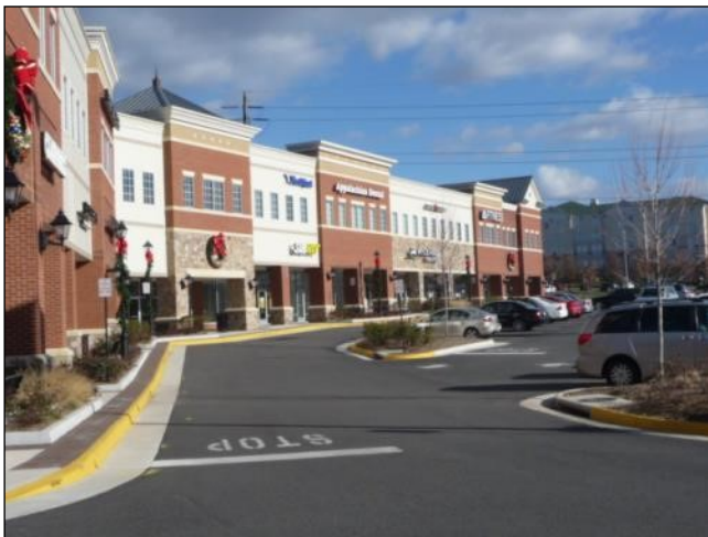
Figure 1117-J: Parapet walls with cornice treatments are used to disguise flat roofs. The image on the right illustrates a tall, thin parapet wall that is prohibited.
